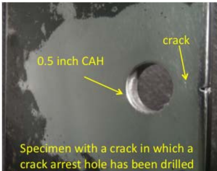
Figure 8. Picture of a CAH Repaired Crack
