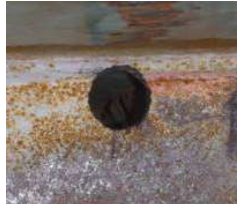
Figure 12. Typical Crack Arrest Hole at End of Weld Crack
