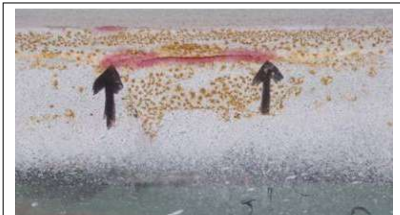
Figure 11. Typical Weldment Crack
