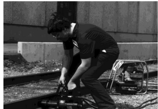
Figure 7. RailTec System in Use on Existing Track
