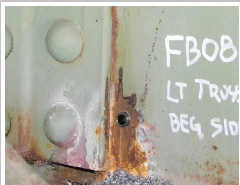
After Repair: StopCrackEX Installed
