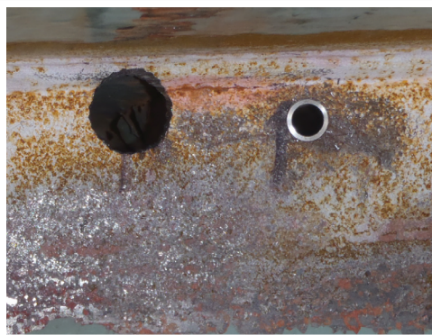
After Repair: StopCrackEX Installed
