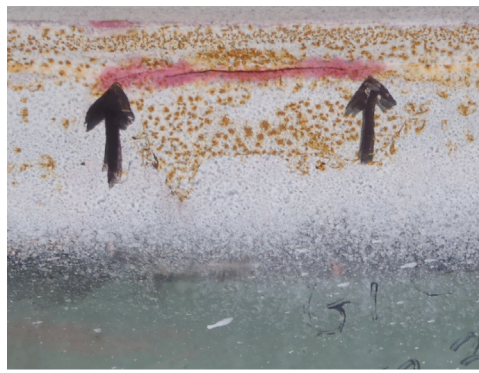
Before Repair: Typical Weld Line Crack
