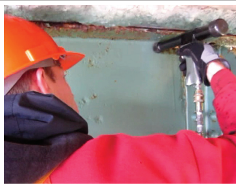
Installing StopCrackEX
