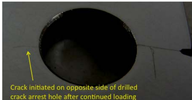
Figure 8: Image of new crack that initiated after being drilled with a crack arrest hole.
