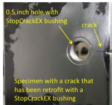
Figure 5: StopCrackEX repaired crack
